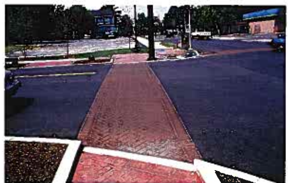
Stamped asphalt crosswalks can provide an aesthetic solution that tolerates snow removal.
